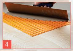
Matting can be levelled immediately with ARDITEX NA, to quickly and easily create a flat, level surface.
