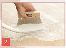
For maximum coverage, spread ARDEX AF 200 PLUS with a B1 or 2mm x 6mm v-notch serrated trowel. When finished, reseal the tub ready for the next job.
