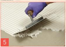
ARDITEX NA can be tiled onto after just 3 hours with an ARDEX Cement-Based Tile Adhesive.
